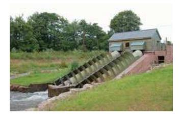
With a fall of one meter in height and a debit(flow) of  $1 \text{ m}^3$ , we can install a unity of a capacity about 7,5 kW.
