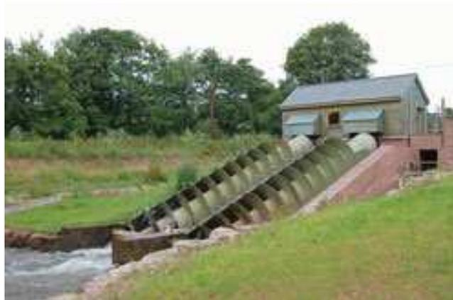
With a fall of one meter in height and a debit(flow) of  $1 \text{ m}^3 /$ , we can install a unity of a capacity about 7,5 kW.
